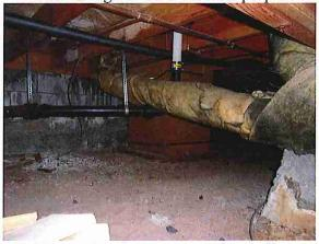
~Evidence of moisture penetration (efflorescence) at the foundation walls throughout with minor to
