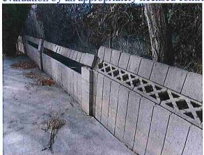
~The gate at the west is displaced/wired shut with loose/unstable block pilaster – does not appear stable at the time of the inspection – recommend further evaluation by an appropriately licensed contractor
