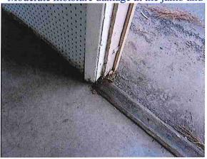
~There is minor to moderate moisture damage at the bottom half of the door with evidence of prior patching/repair – dry at the time of the inspection
