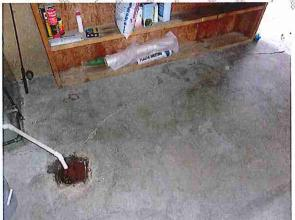
~There is a crack of 1/4" or larger that runs across the floor at the northeast – needs sealant/repair
